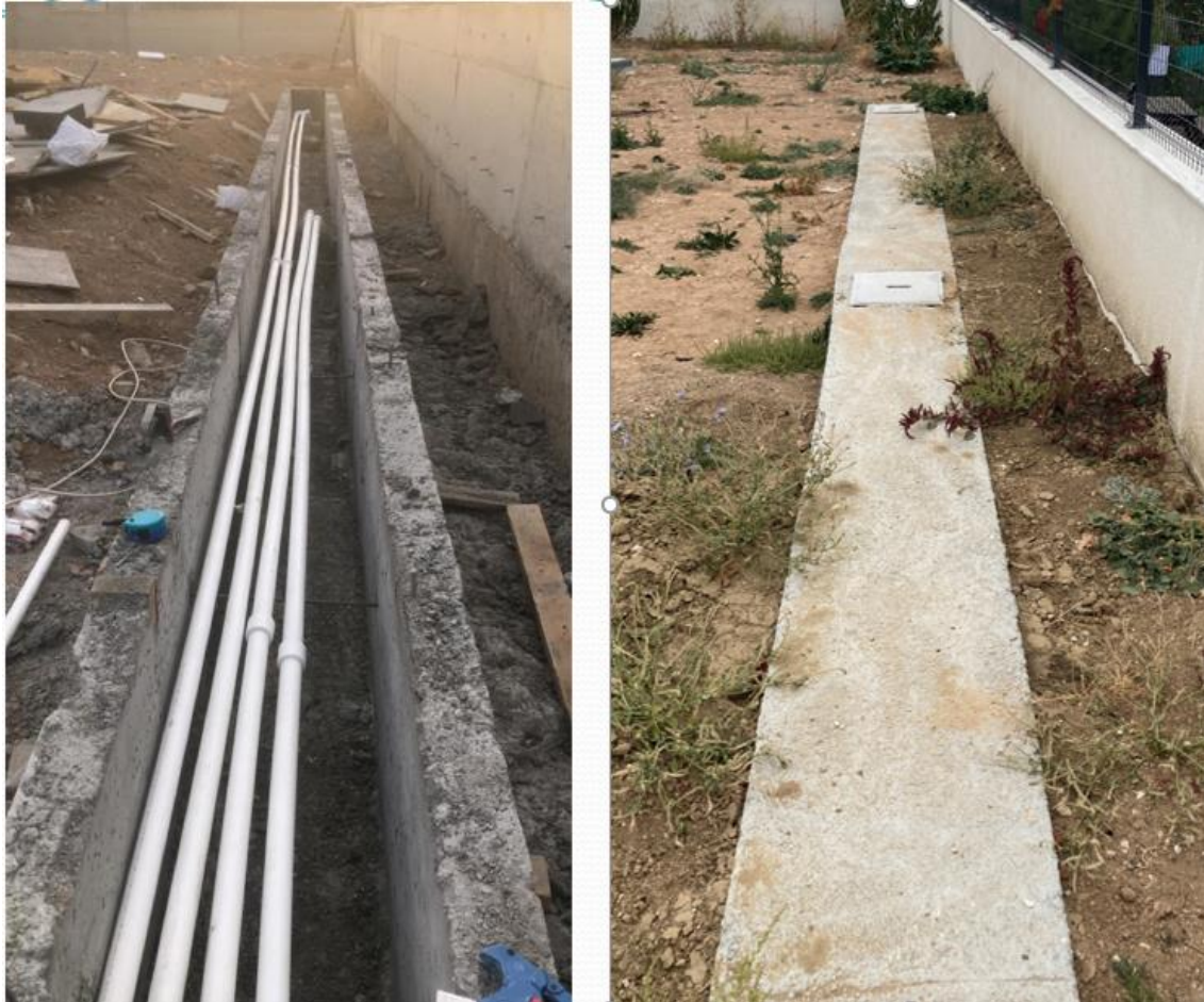
248 Figure 5 BHE concrete canal application
